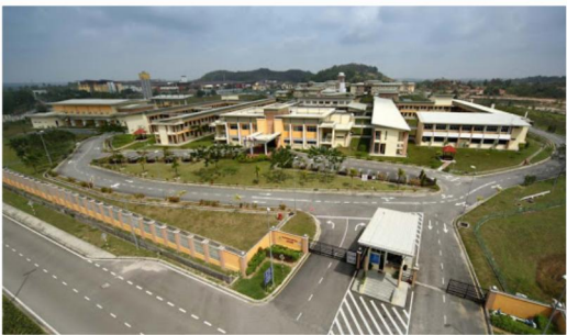
Proposed construction of a 100 ft road leading into MRSM Bandar Seri Alam, Johor Bahru. Earthworks computation, design of external sewer line and external water reticulation leading to the reservoir.
