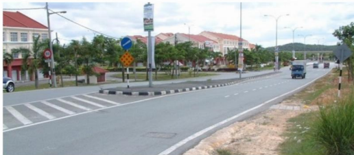
JKR Road J4 (Package B11) Jalan Lima Kedai/Gelang Patah road upgrading.
