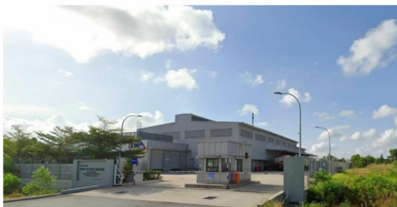
DDW Colours factory designed to produce caramel for Coca-Cola and Pepsi (architectural, civil infrastructural and structural design).
