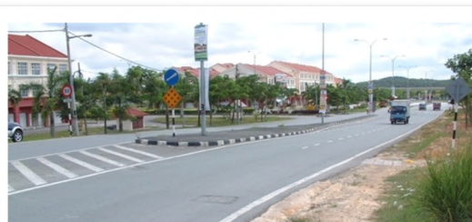
JKR Road J4 (Package B11) Jalan Lima Kedai/Gelang Patah road upgrading.
